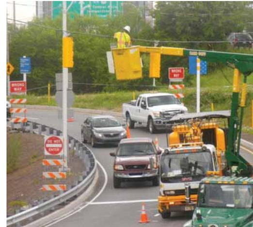
*Workers install temporary signals at Girard Avenue and Aramingo Avenue north to provide access to the reopened northbound on-ramp.*
