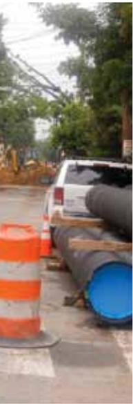
*Installation of a new gas main on Edgemont Street: PennDOT is providing new gas, water and sewer mains beneath a number of surface streets near the Girard Avenue Interchange.*
