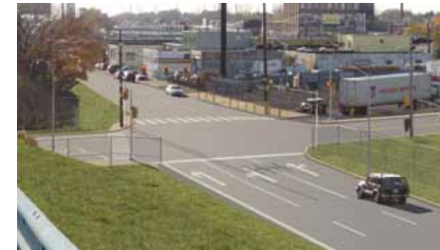
CP2 improvements include reconstruction of the southbound ramp and intersection at Bleigh Avenue, as shown in this rendering.
