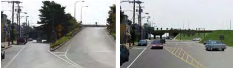
Above: Princeton Avenue with and without the southbound on-ramp. The Princeton Avenue ramp is being replaced by the State Road on-ramp (below).
