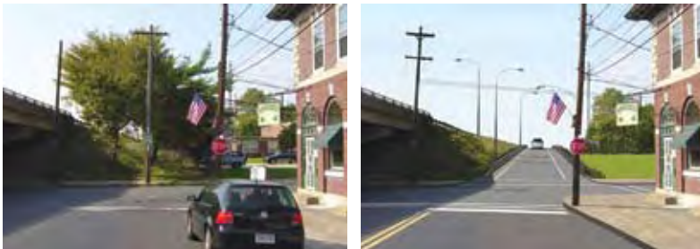
Above : State Road without and with the new southbound on-ramp to I-95
